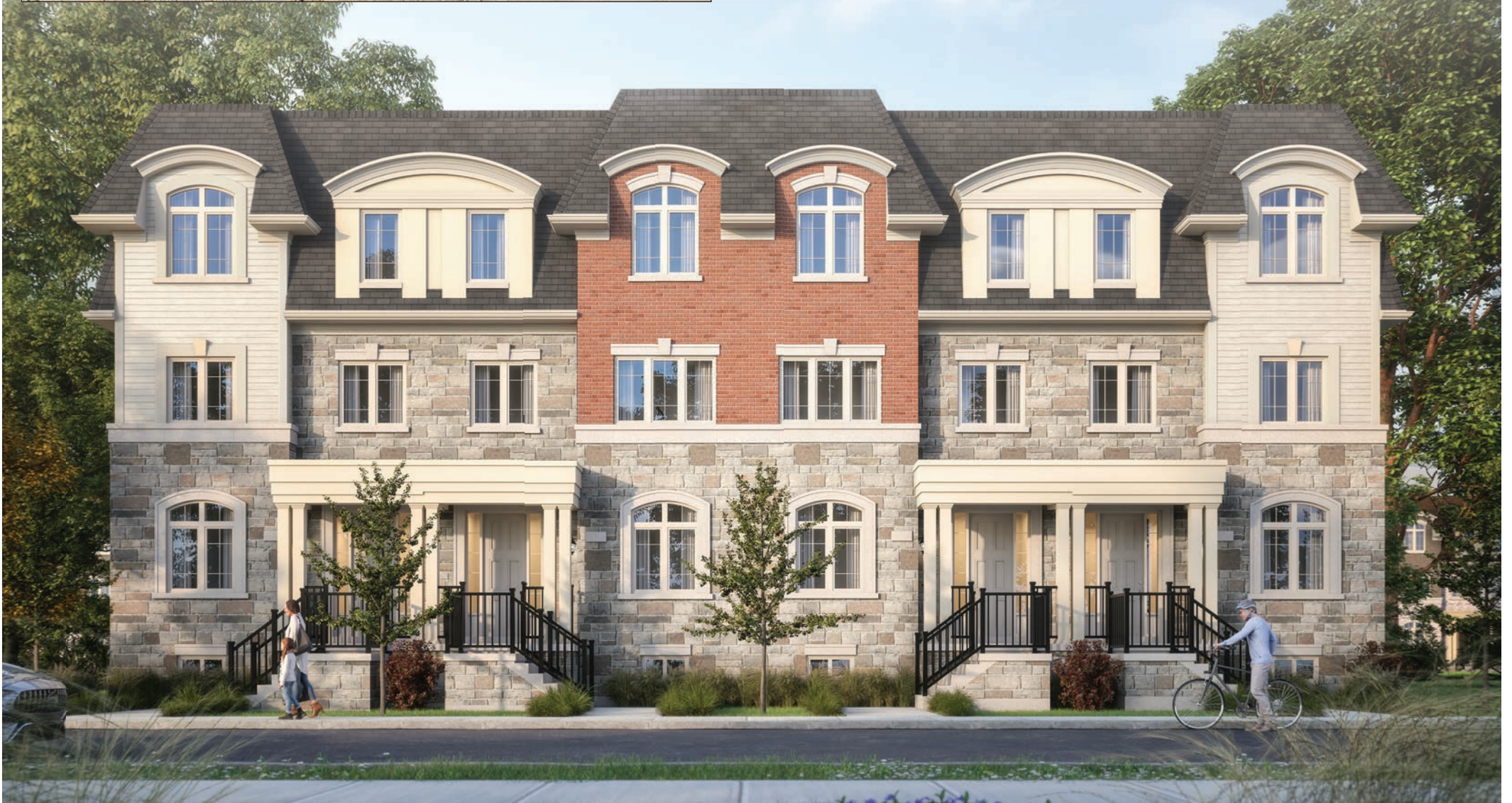
The shovels went in the ground to launch the King City luxury townhouse project by Camcos. Shown are (l to r) James Circosta, Mike Circosta, Mayor Steve Pellegrini and Nino Campoli.
